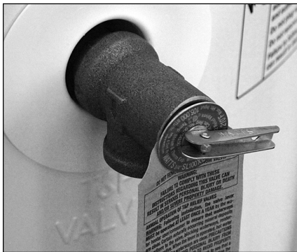
Figure 25 - Temperature and Pressure Relief Valve
