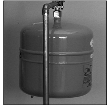
Figure 29 - The Thermal Expansion Tank should be pressurized with air, using a hand pump, to match the home's incoming water pressure.
