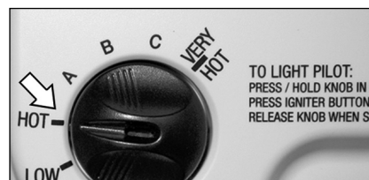
Figure 36 - Adjust the gas control knob to "HOT".
