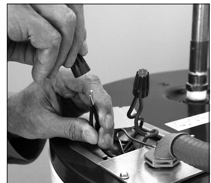
Figure 19 - Connecting the electrical wires.
