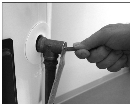
Figure 38 - T&P Relief Valve
