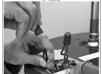
Connecting the electrical wires.
